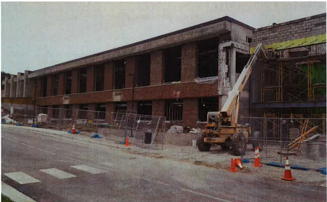
Window openings, masonry & steel @ east elevation
