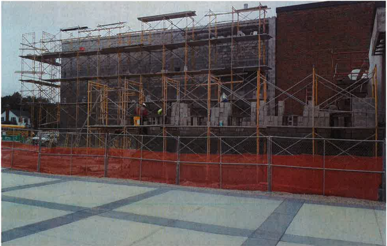
Window openings, masonry & steel @ east elevation
