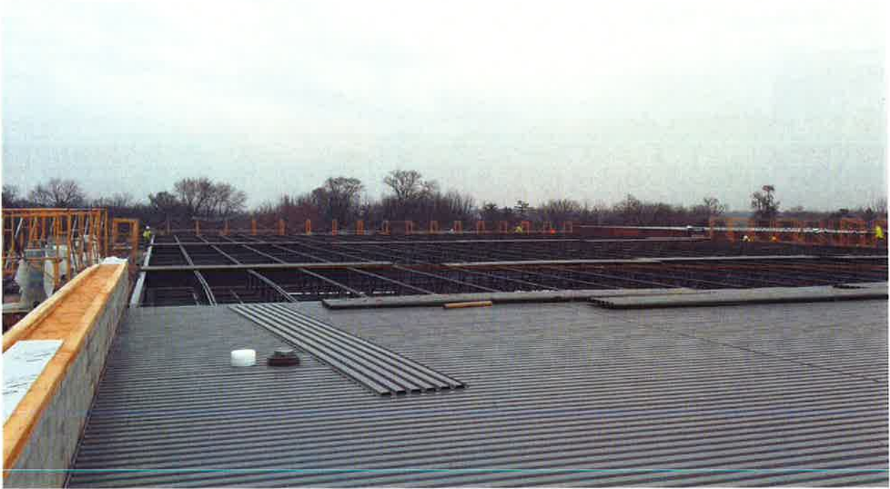
Installing roof deck
