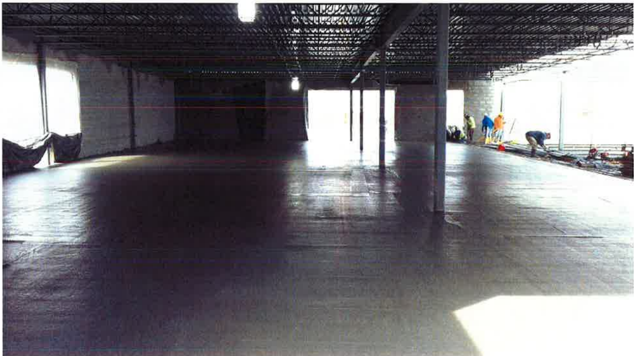
Pouring of 2 nd floor slab
