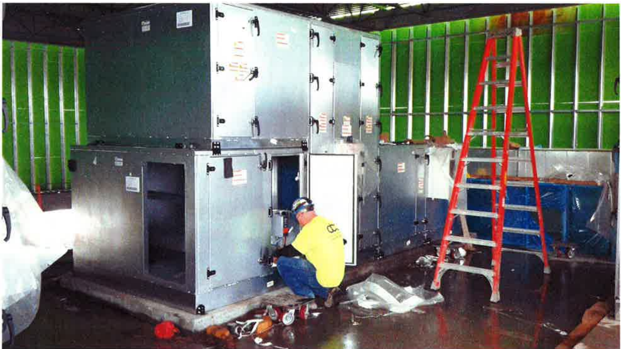
HVAC units being installed in mechanical penthouse
