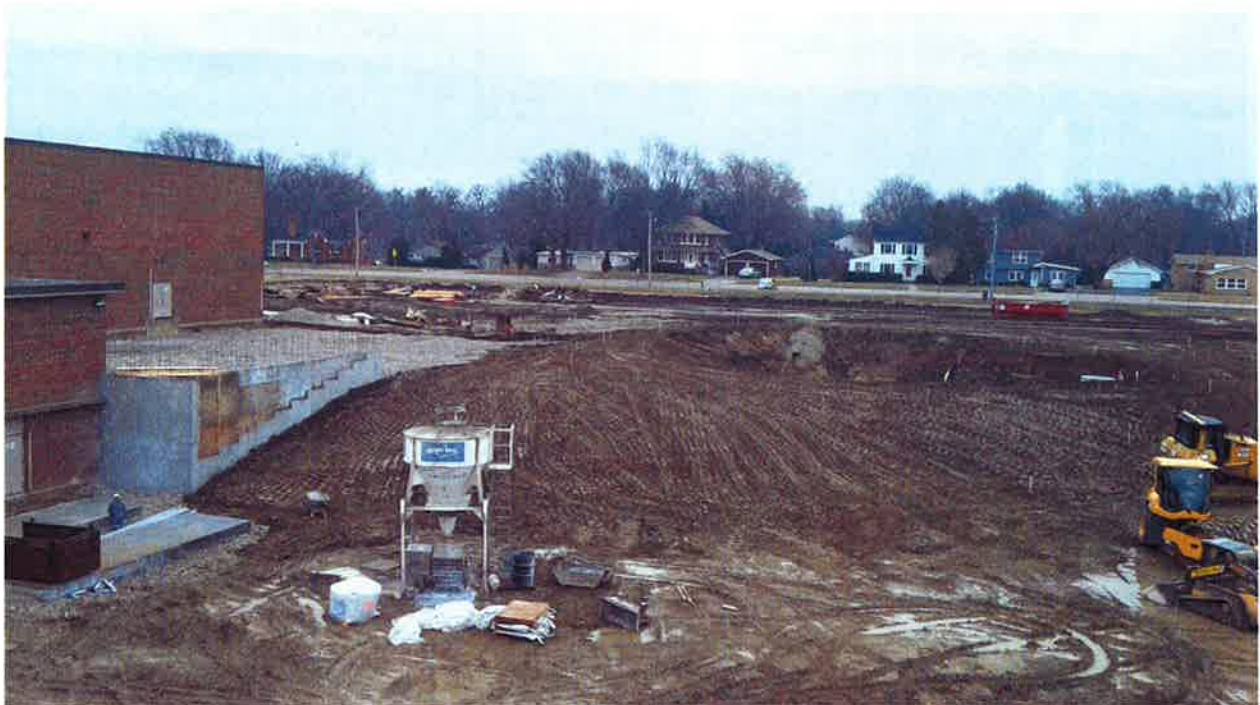
Rough grading of parking, slope and detention
