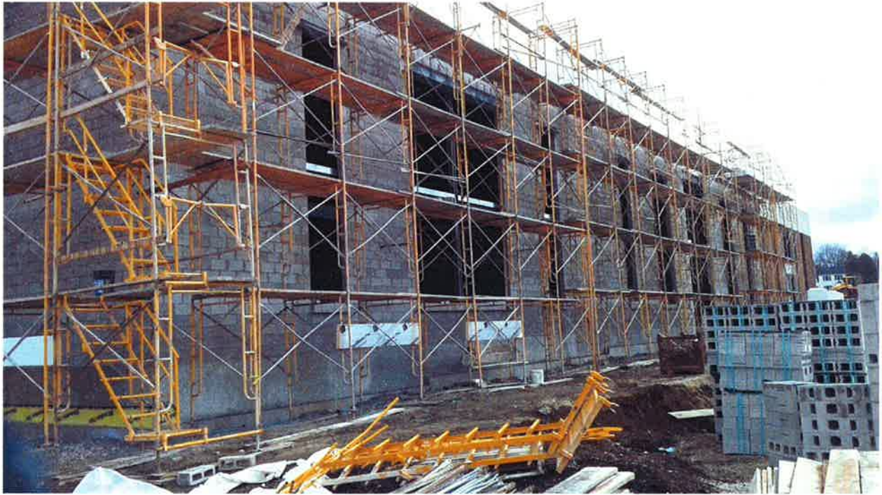
Masonry block to top of wall height
