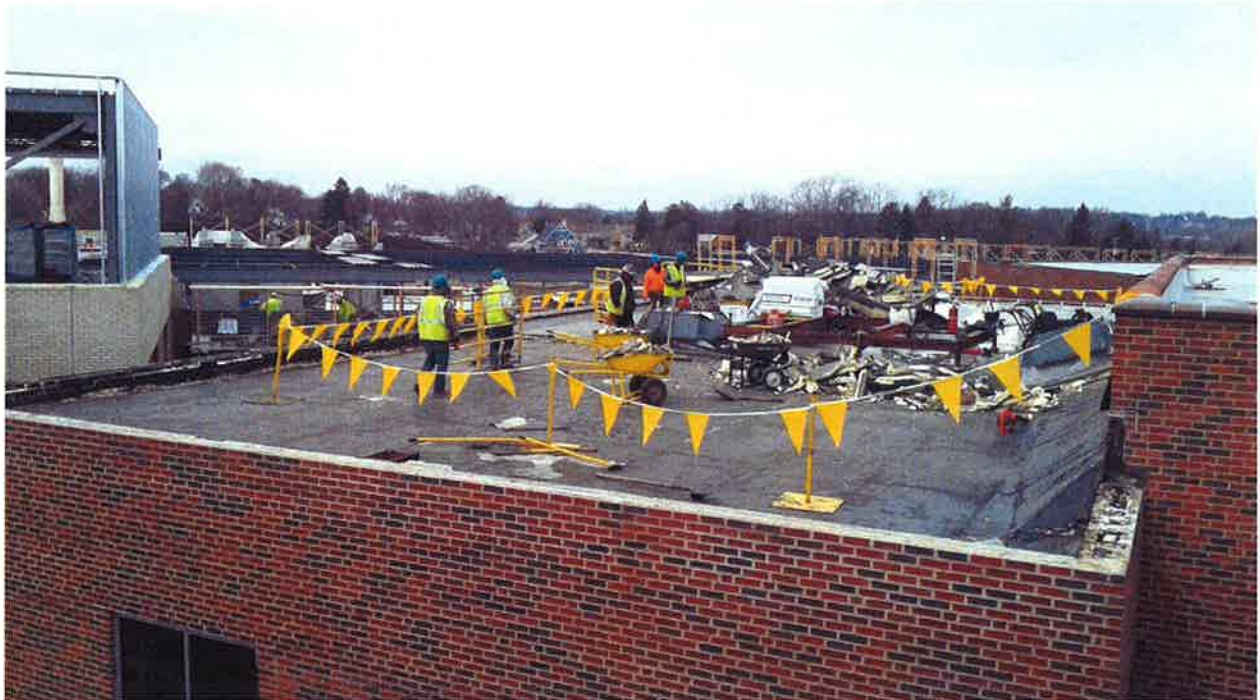
Removal of existing roofing
