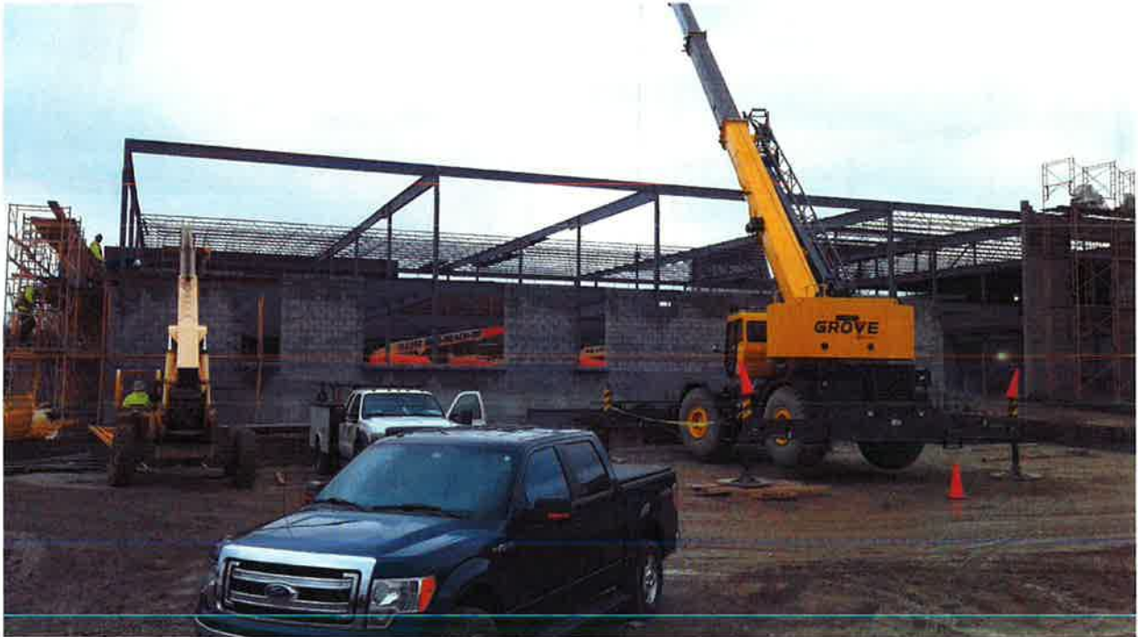
Structural steel & masonry
