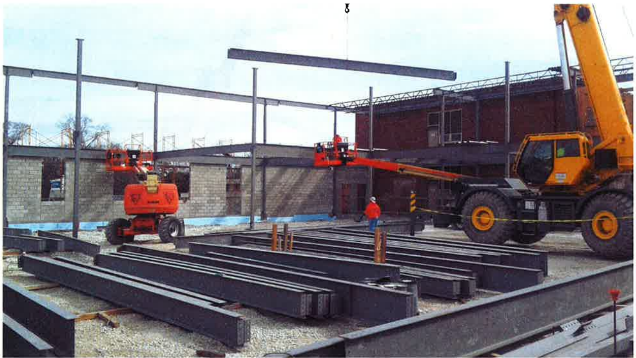
Classroom addition structural steel installation 3/26/18
