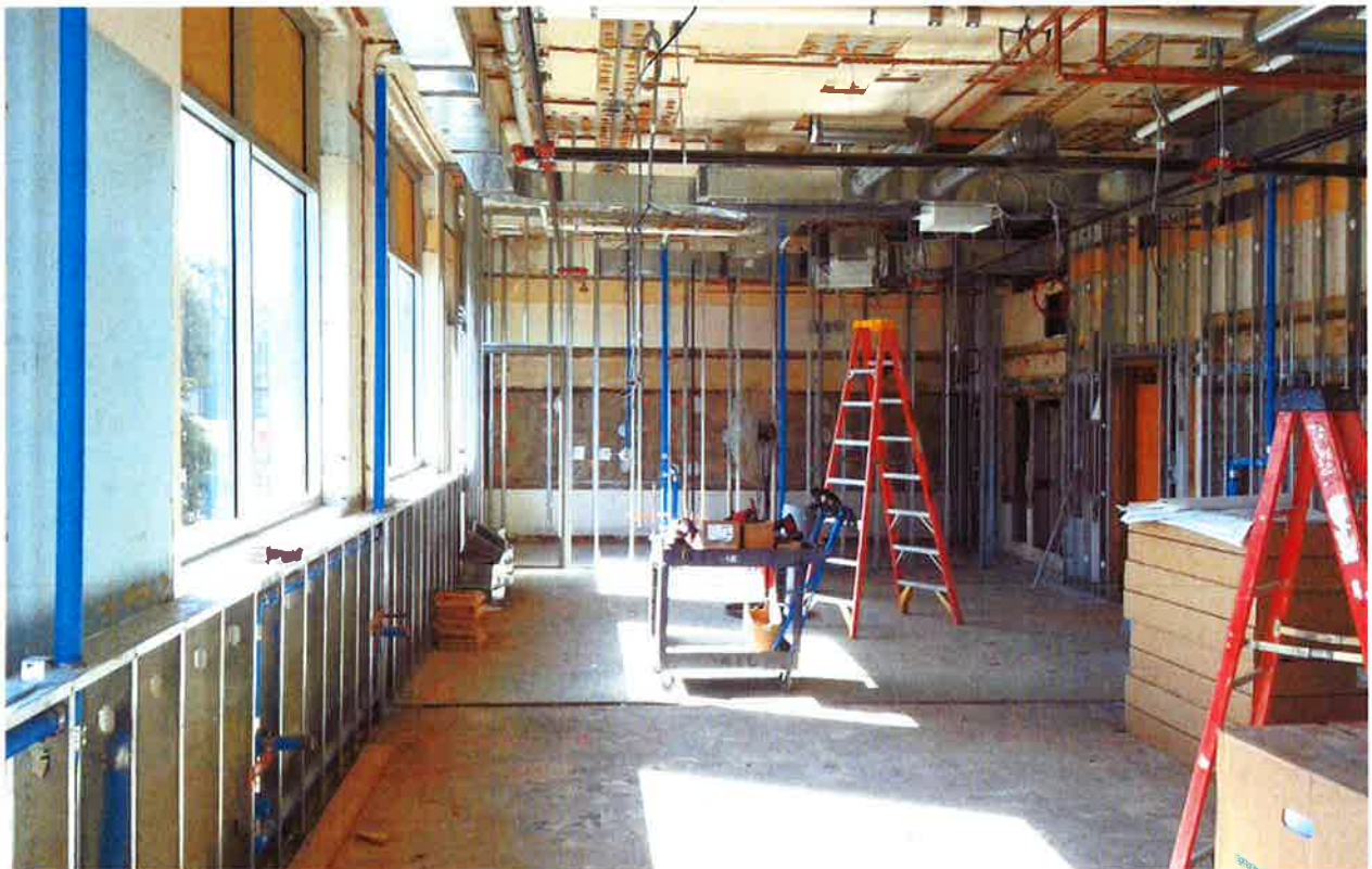
Interior framing and MEP rough in
