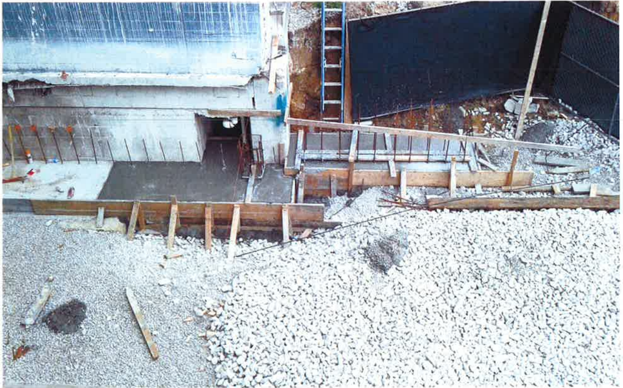
Foundation wall framing new entrance
