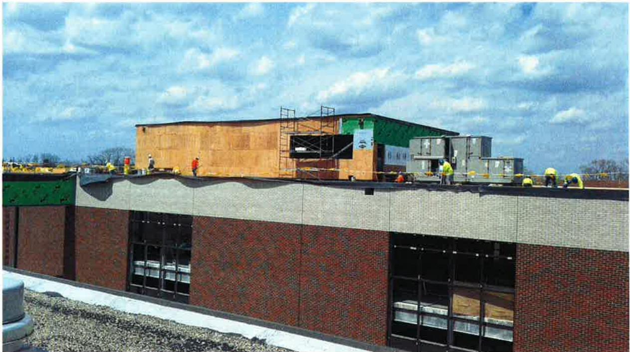
Mechanical mezzanine sheathing
