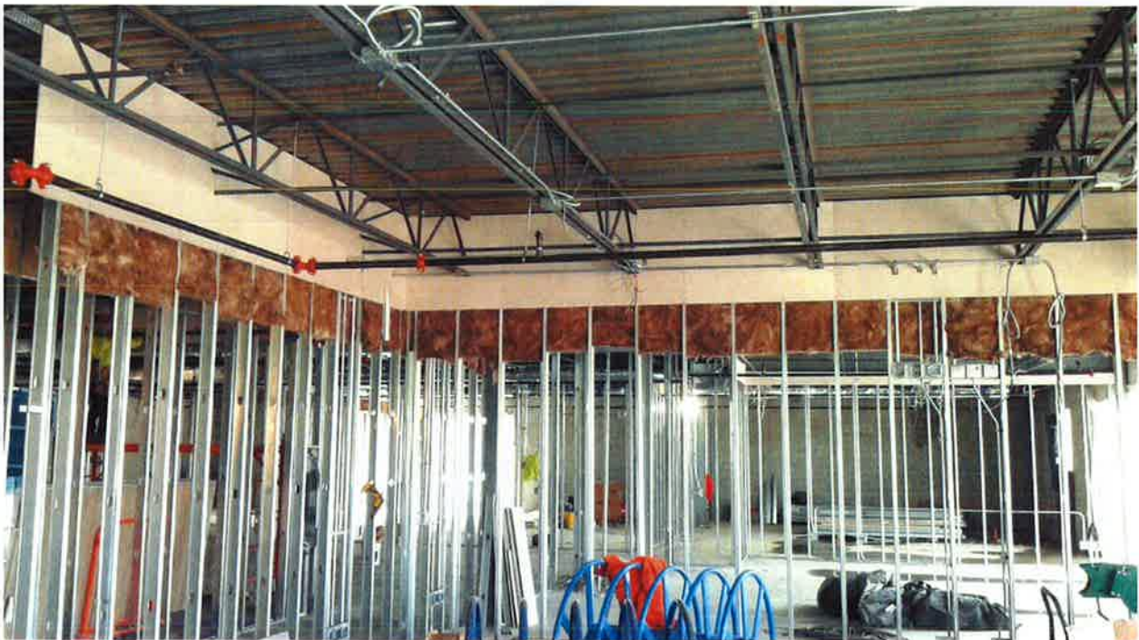
Wall framing, drywall install 2 nd floor classroom addition
