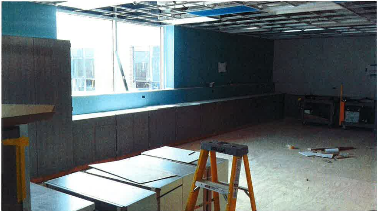
Science casework, subfloor complete, ceiling grid & light fixtures set
