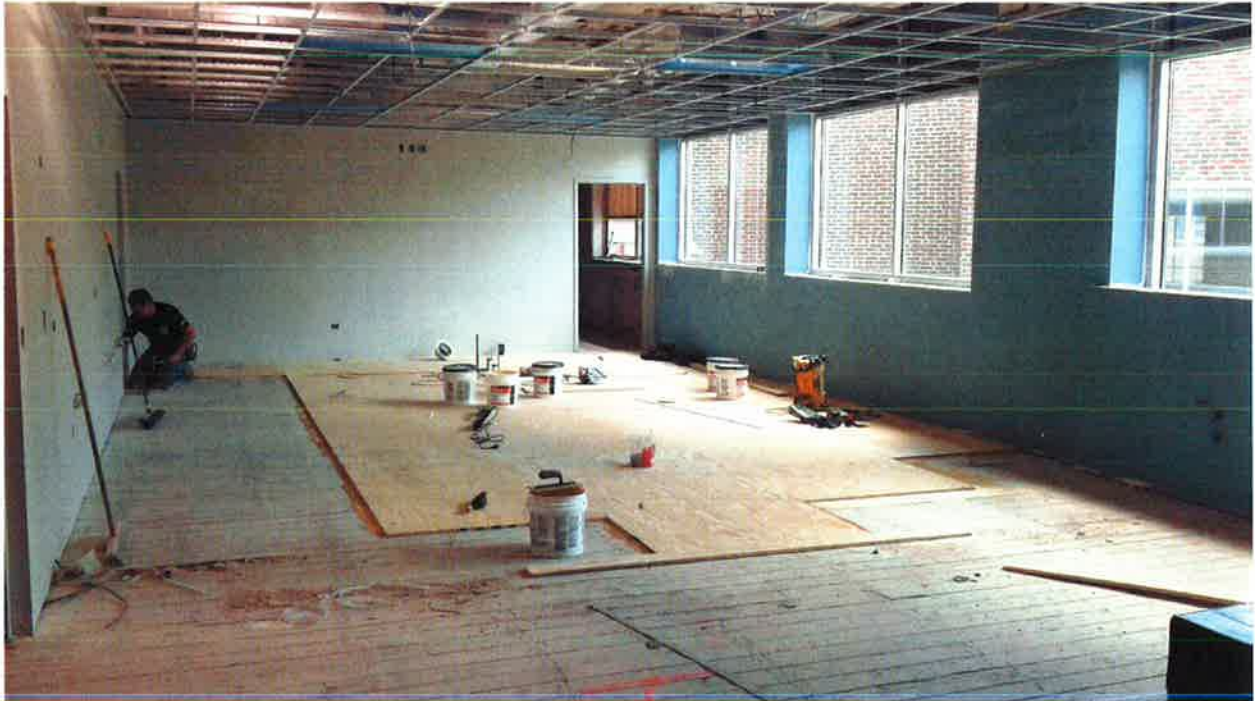
Underlayment installation
