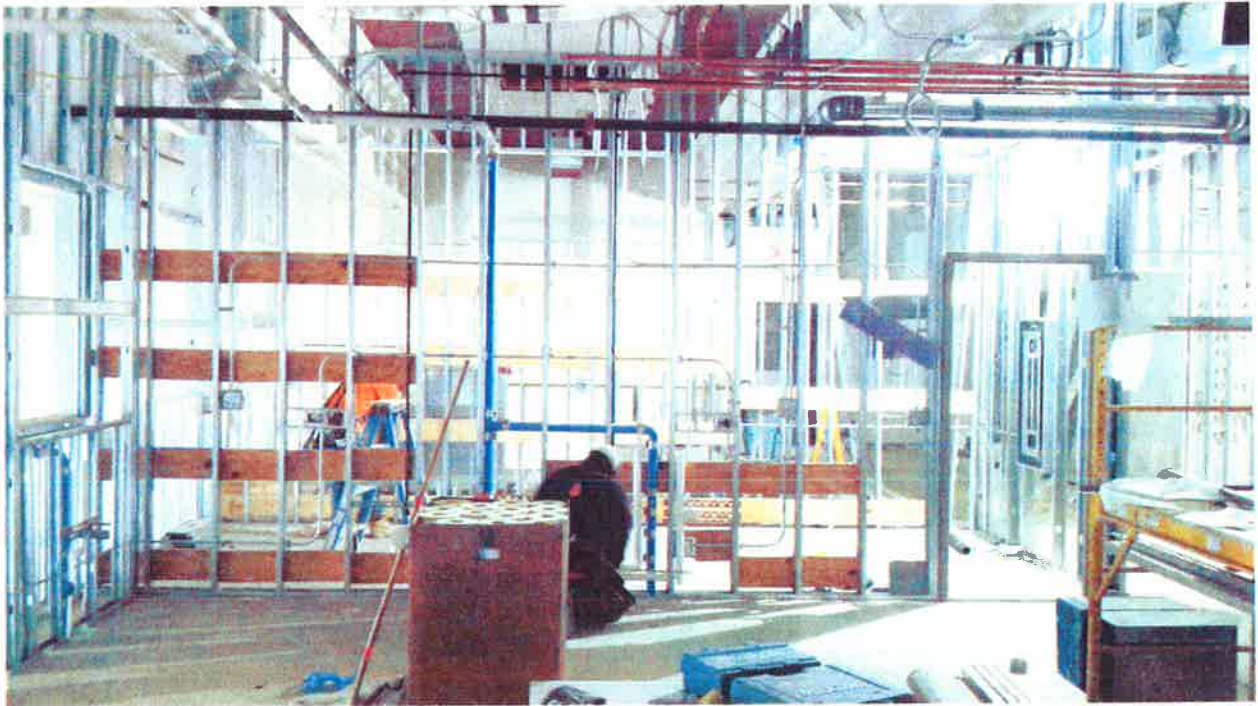
Wall framing & wood blocking @ Science and Prep Room
