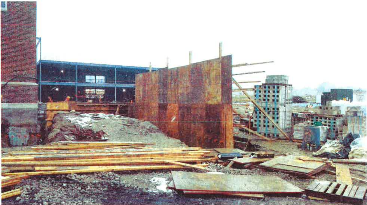
Loading dock retaining wall framing
