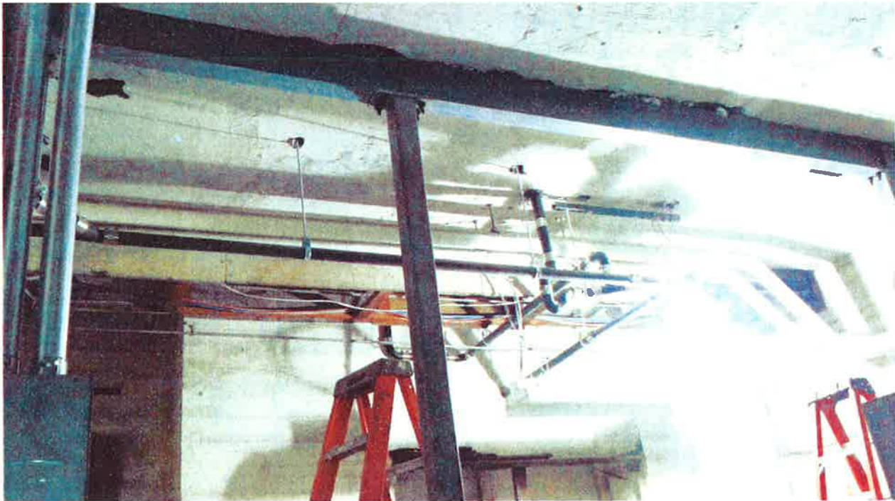
Interior steel installed to support Kitchen area
