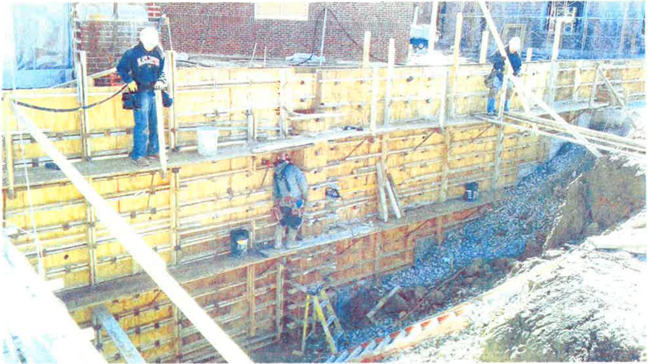
Last interior courtyard foundation wall forming
