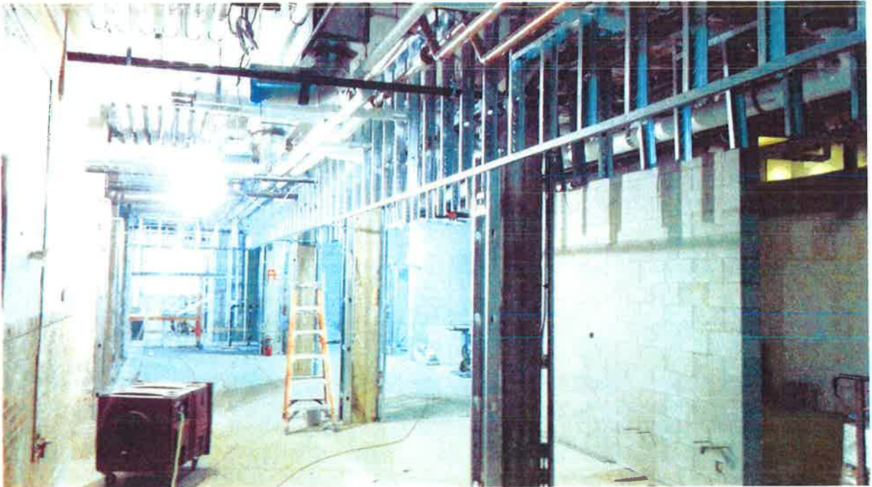
Kitchen area soffit framing
