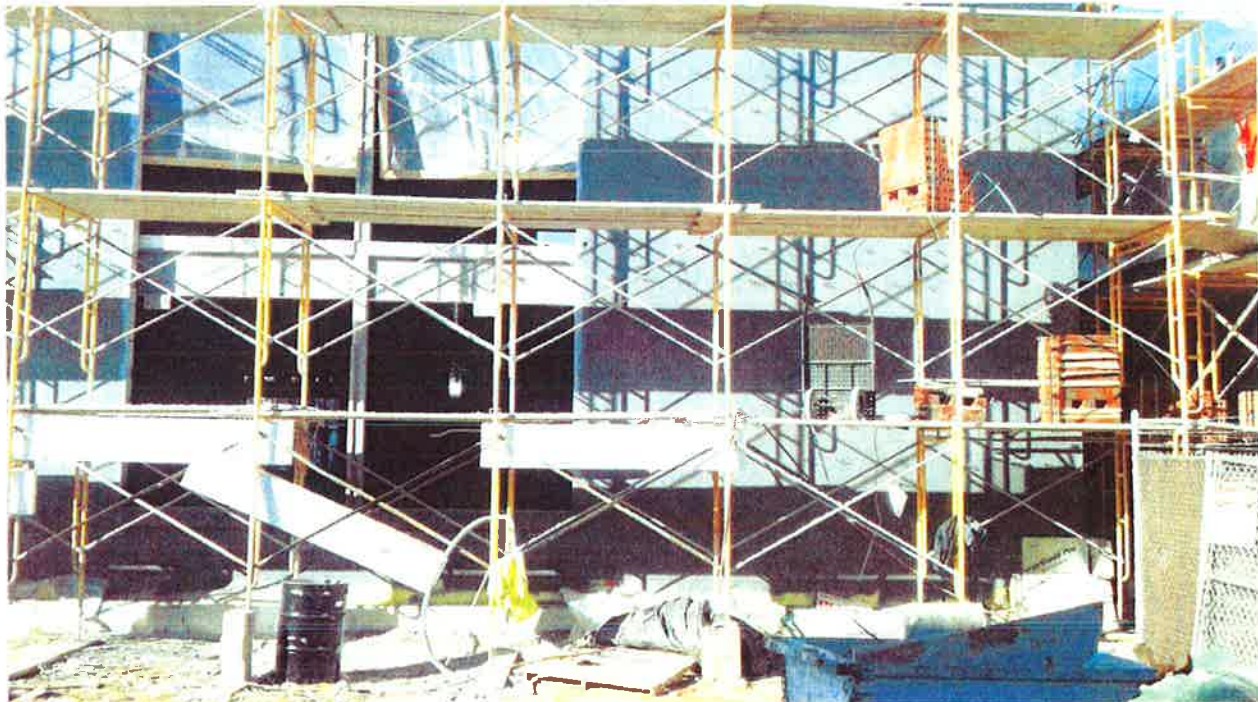
Air barrier installed, ready for insulation & brick 2/27/18
