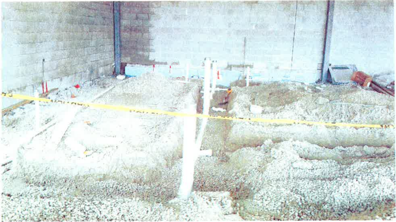
Underground plumbing in addition
