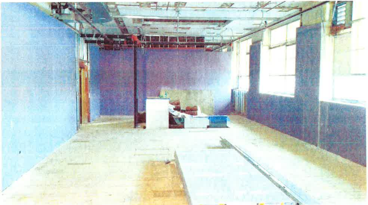
Abuse resistant drywall installation in classroom
