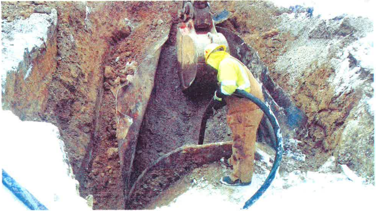
Removal of discovered unknown underground storage tank
