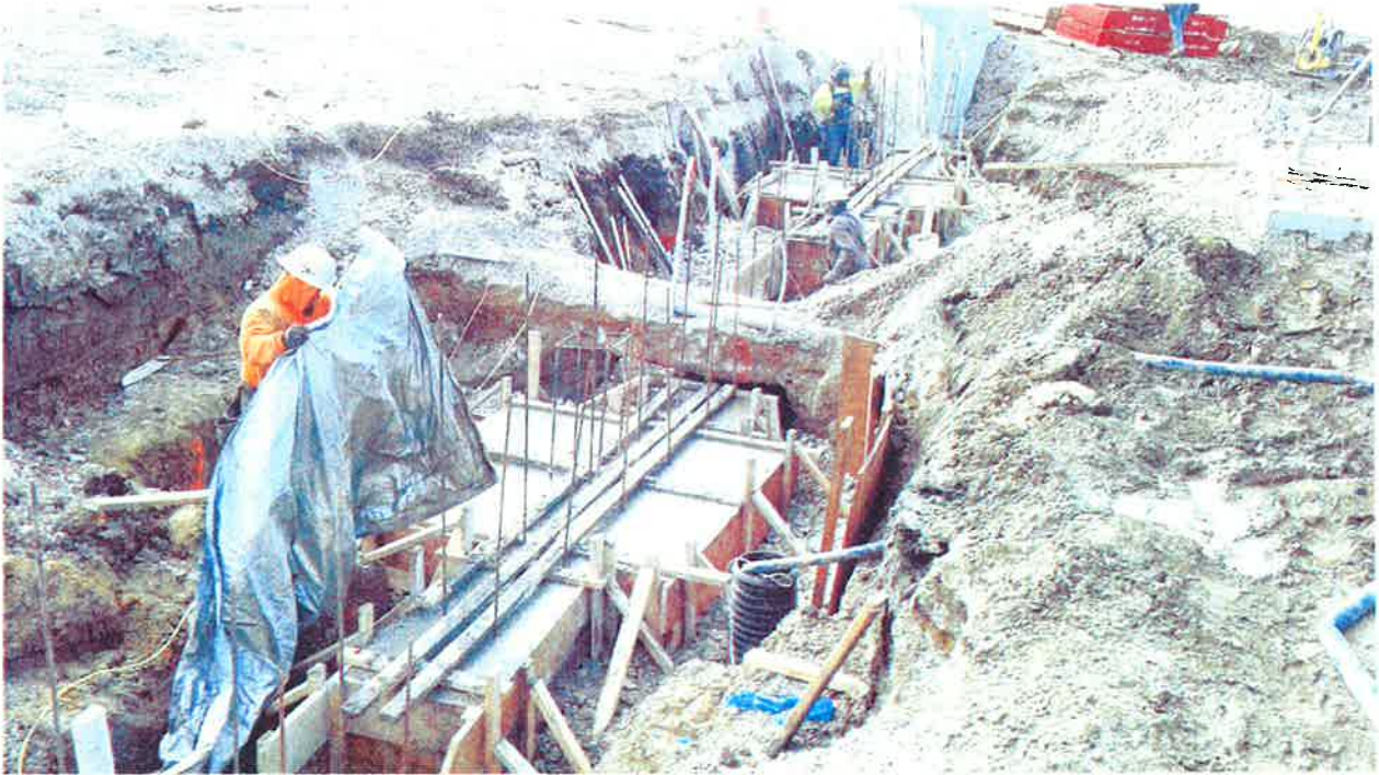
Final footing for addition poured
