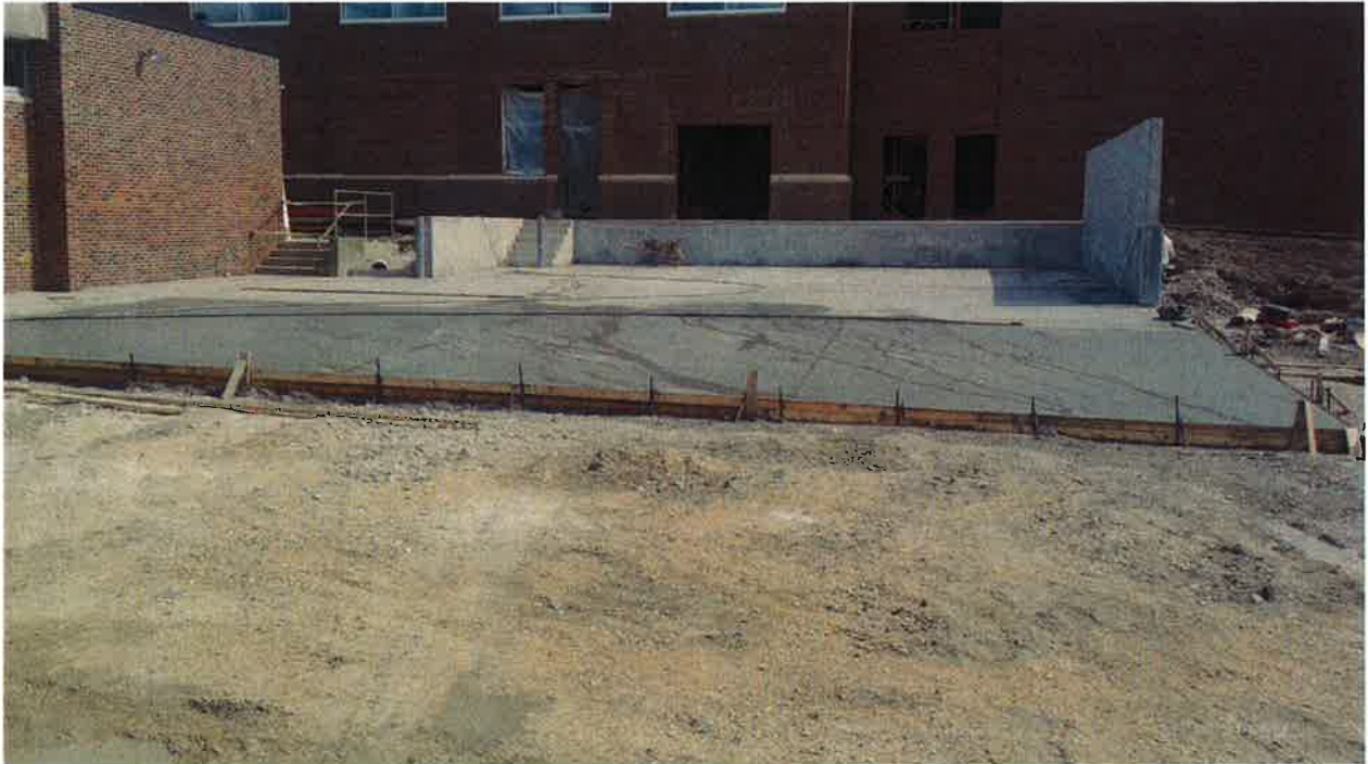
Loading dock concrete complete 5/31/18
