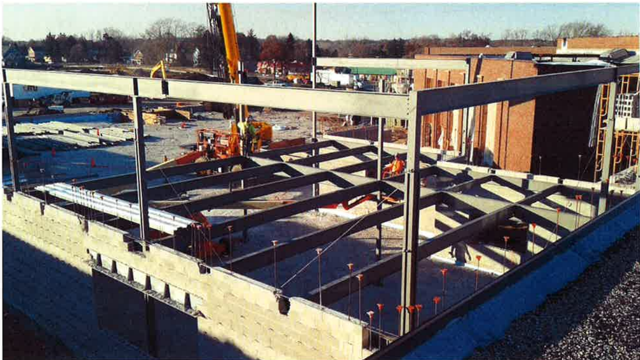
Start of structural steel erection
