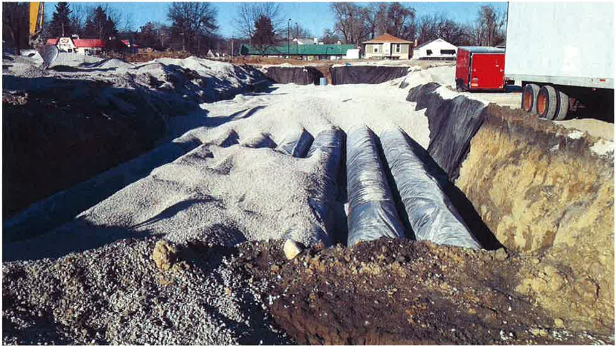
U.G. storm water detention pond #2
