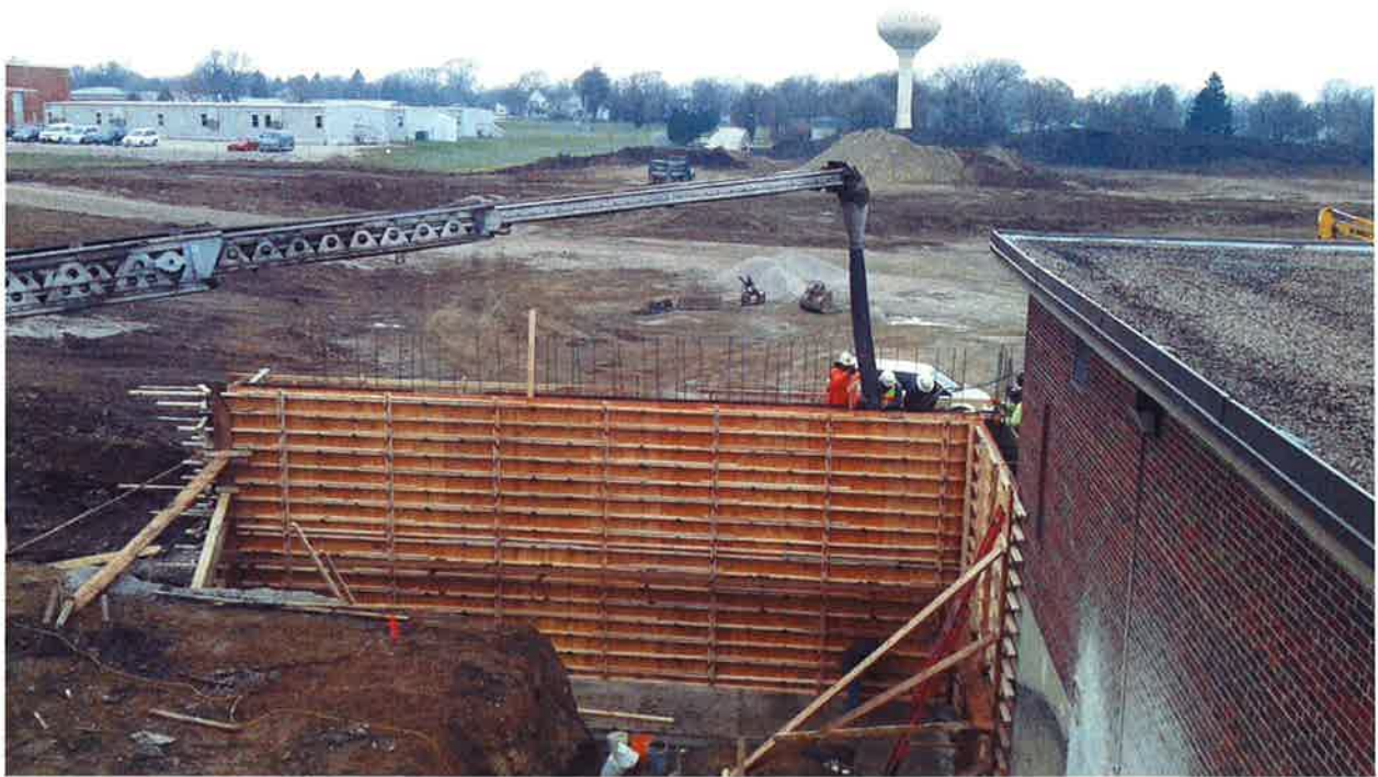
Pouring locker room retaining wall
