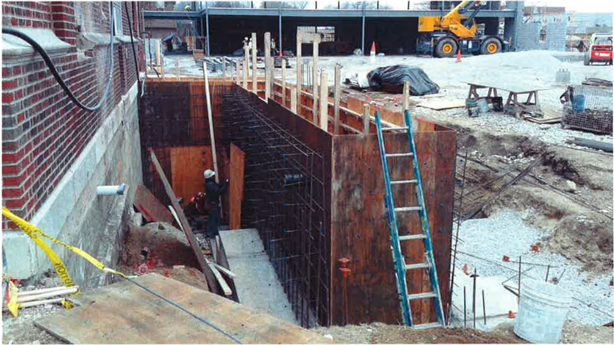
Stair foundation framing at existing/new connection
