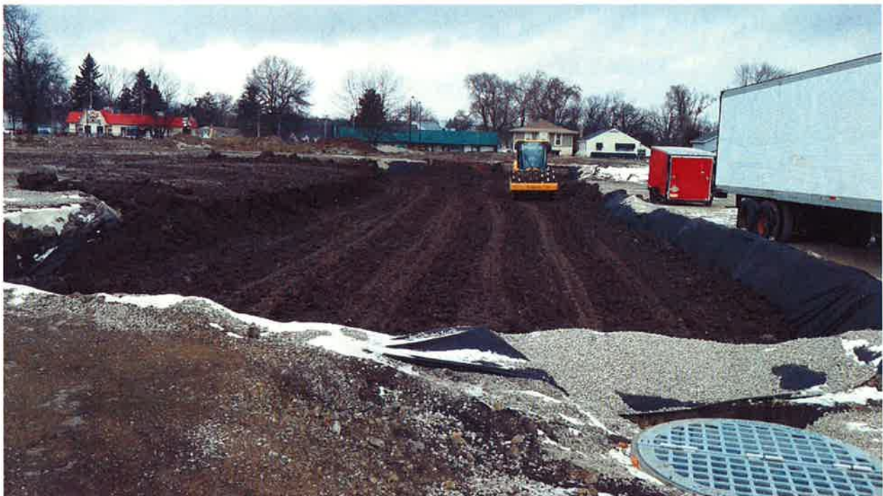
Backfilling U.G. storm water detention pond #2
