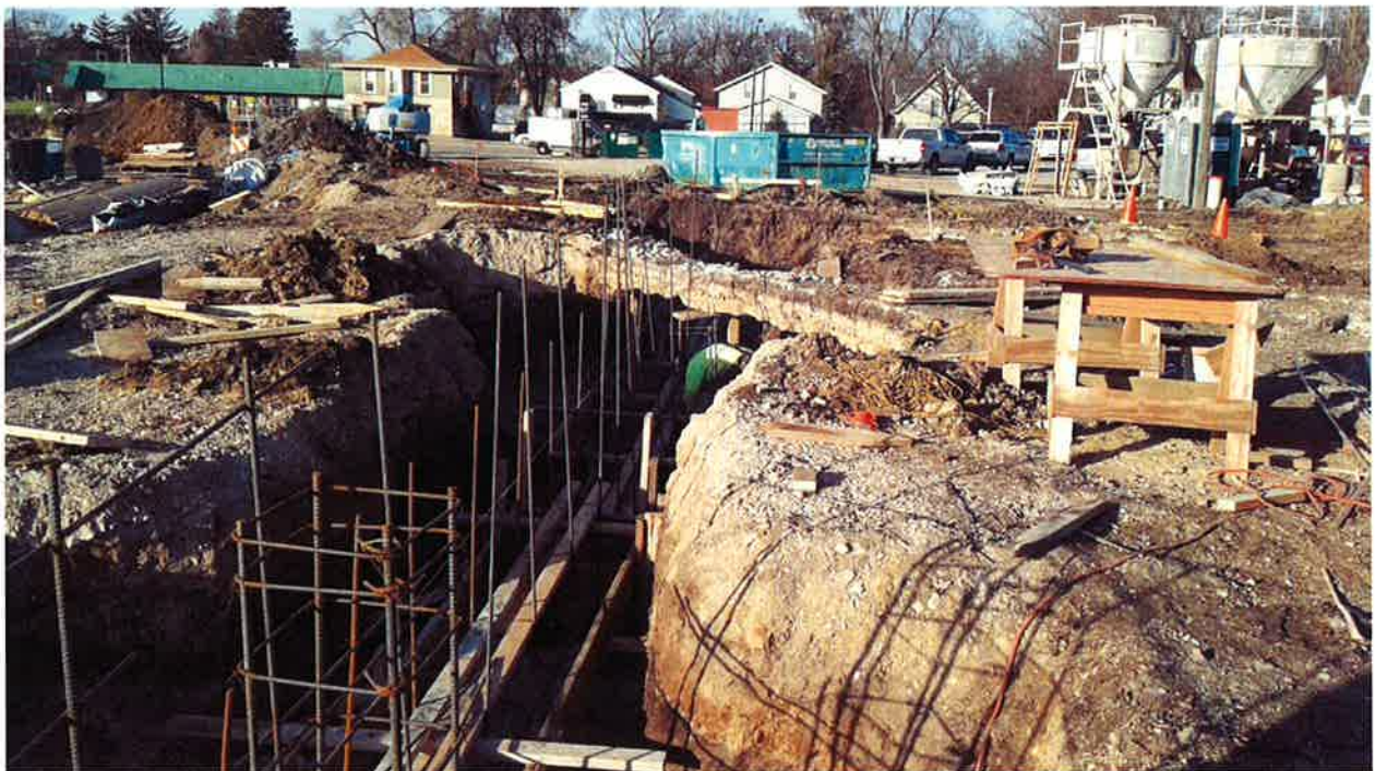
Forming of foundation with electric service running through
