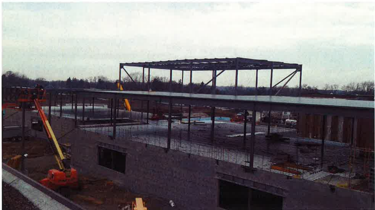
Floor and roof deck installation
