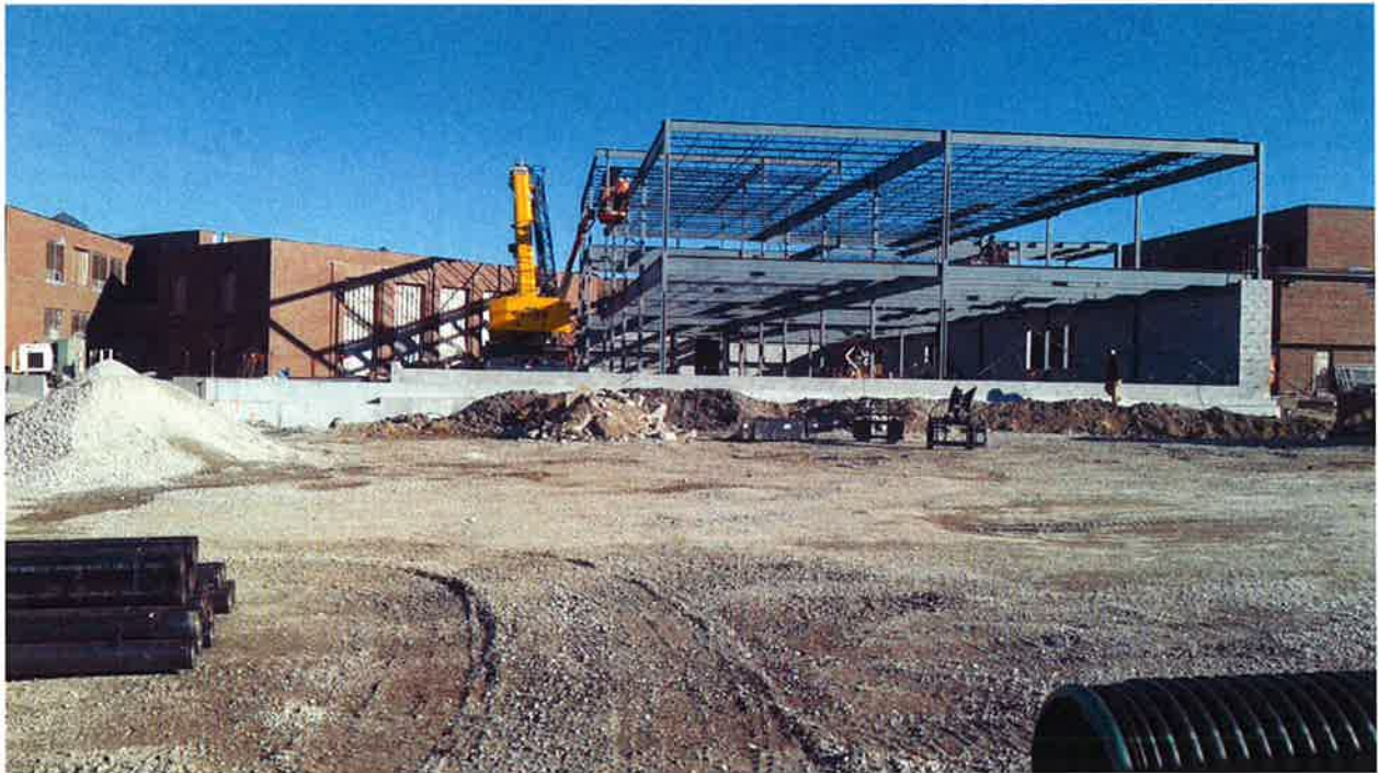
Structural steel joist erection
