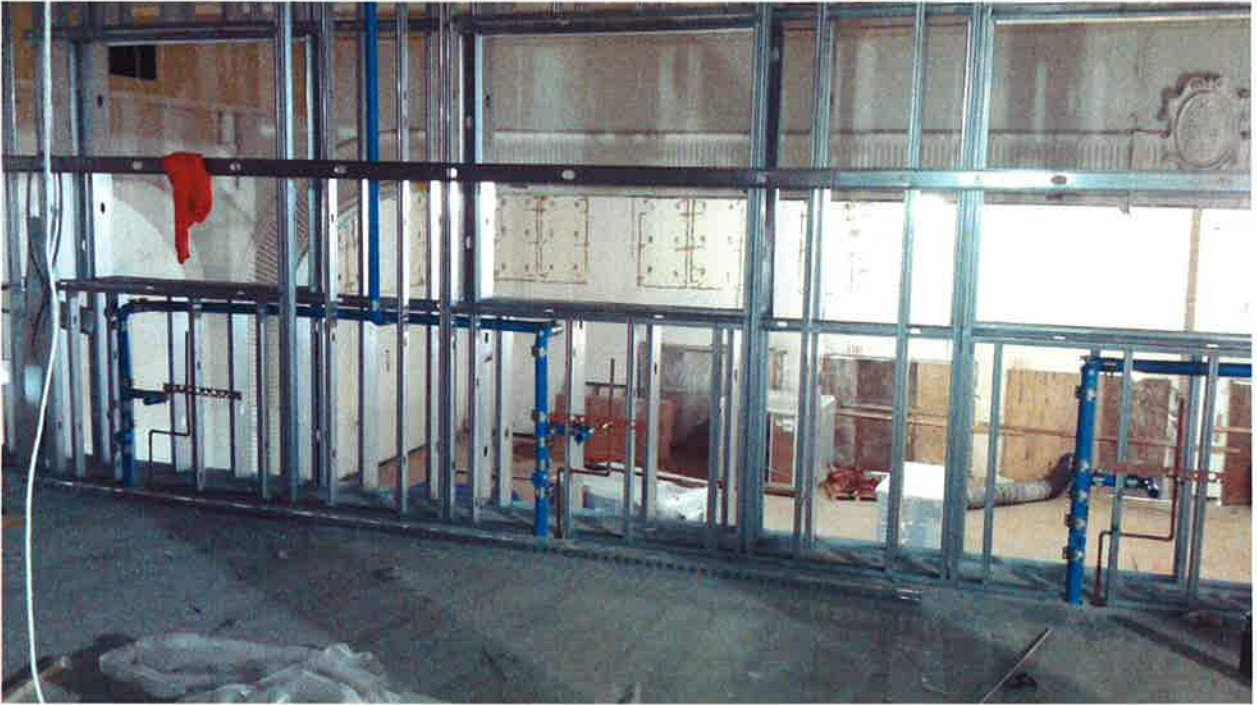
Science room wall framing and plumbing rough-in
