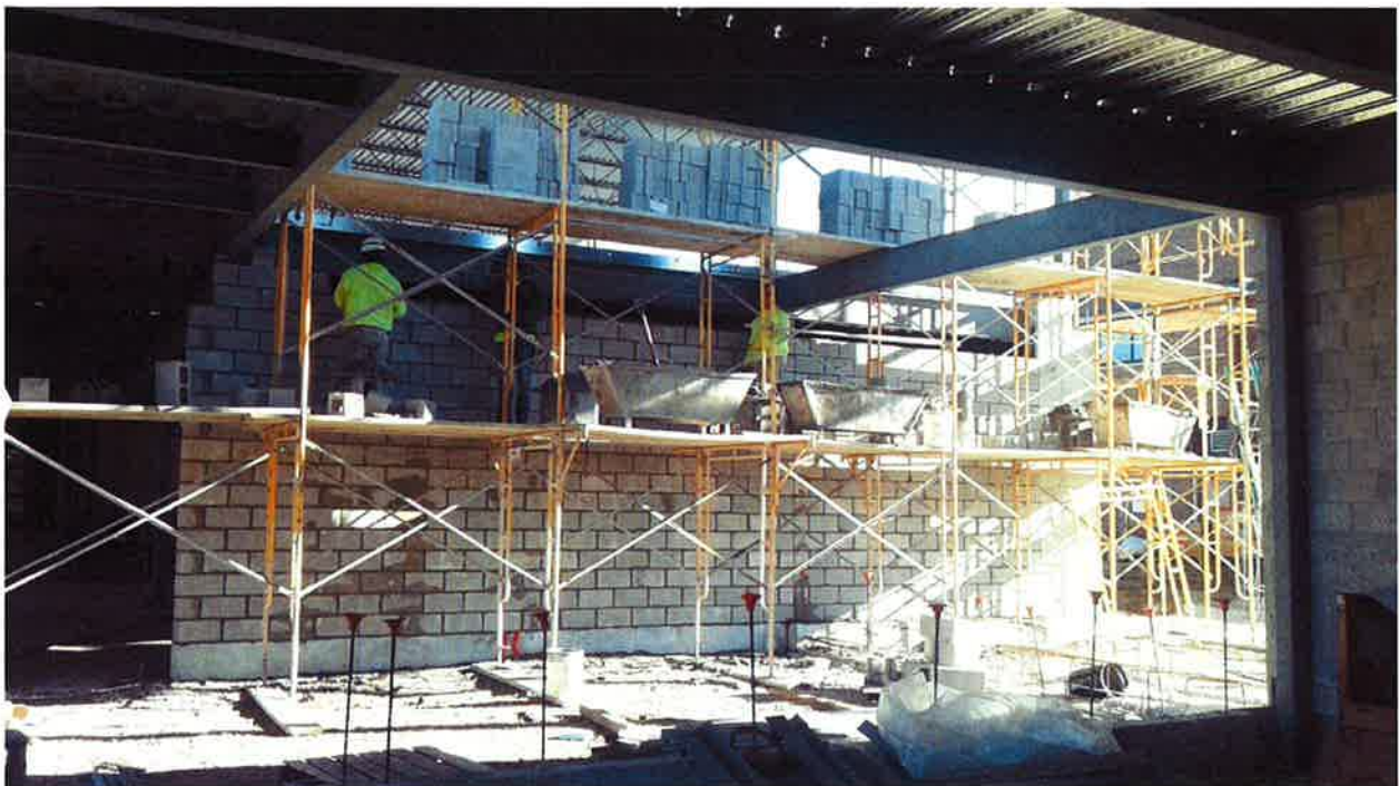
Student entry masonry installation
