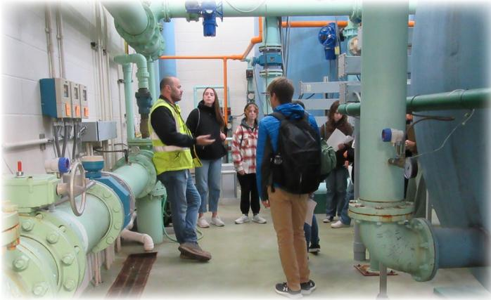
Students from AP Environmental Science and Environmental Science classes observed how the water pumped out of the aquifer is treated for hardness and radium before being distributed to the community. The minerals associated with water hardness and radium are naturally occurring in the rock formation that is the aquifer from which we draw our drinking water.
