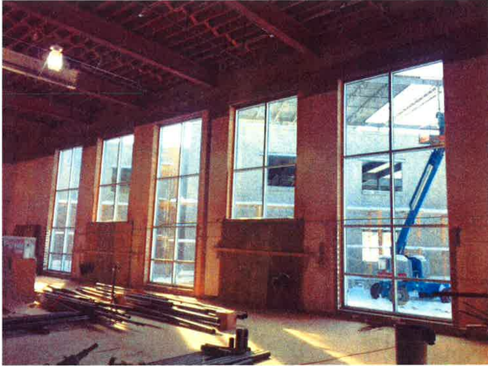
Cafeteria Windows Installed - Interior
