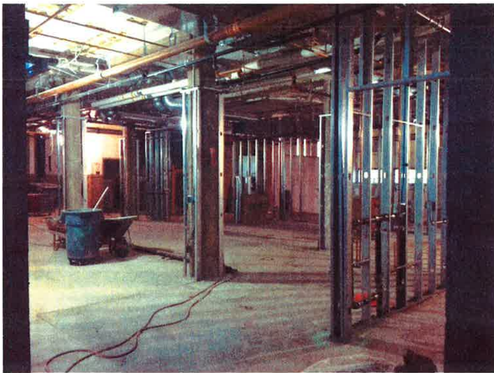
Kitchen masonry and plumbing rough-in (from loading dock entry)
